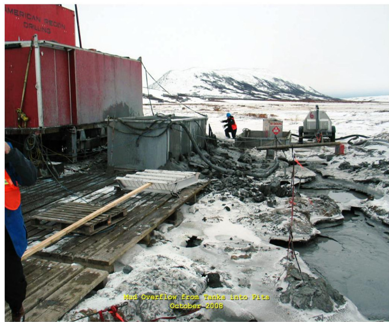
Mud Overflow from Tanks into Pits, October 2008 Source: Department of Natural Resources/State of Alaska
