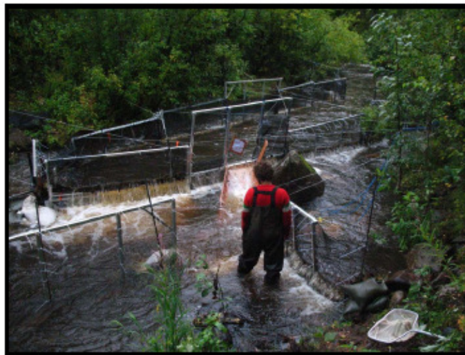
Photo 7. The Stream 2003 ramp for adult salmon traveling upstream being inspected on September 3, 2008. Water flow is from top right to bottom left.
