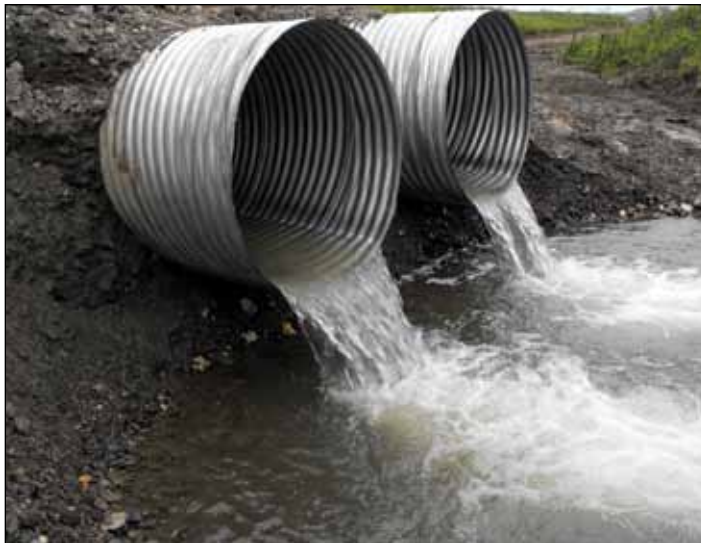
Storm water runoff pouring through these culverts near Rock Creek Mine makes clear the source of excessive turbidity in Lindblom Creek © Derrick Leedy
